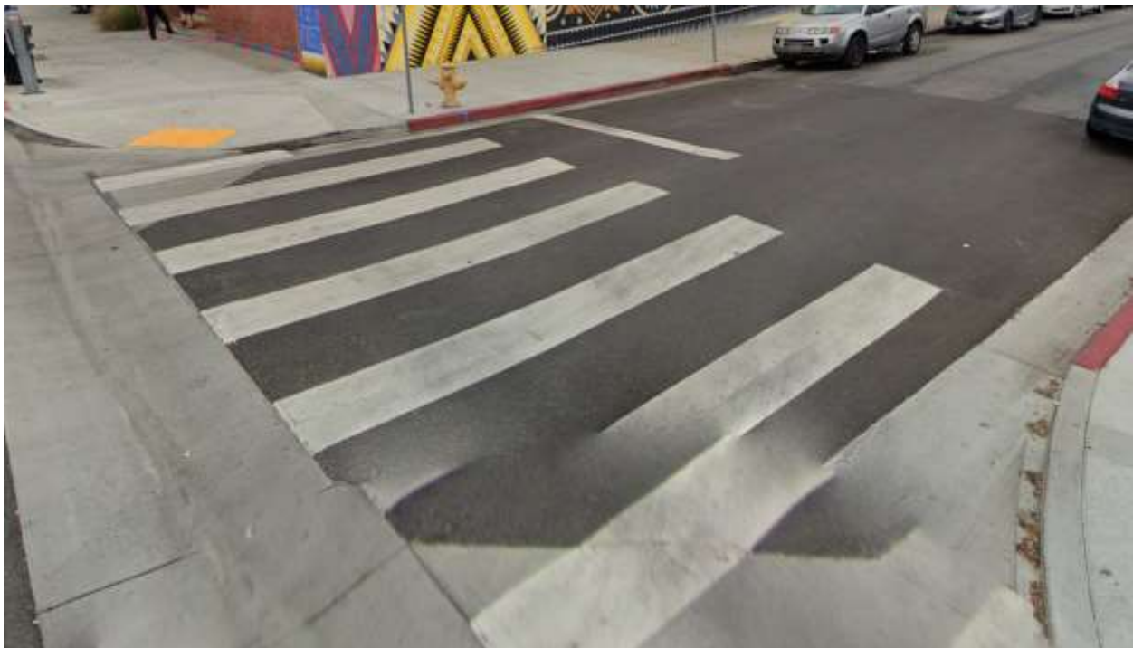
Example of an ADA-compliant curb ramp, high-visibility crosswalk, and advanced stop bar
