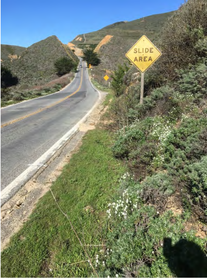
Photo 5: Road shoulder, east side of State Route 1, north aspect (2/7/2018).
