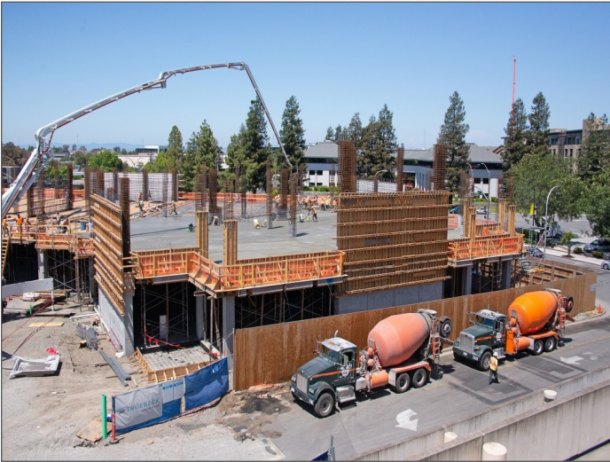
Construction of County Center Parking Structure 2 © County of San Mateo
