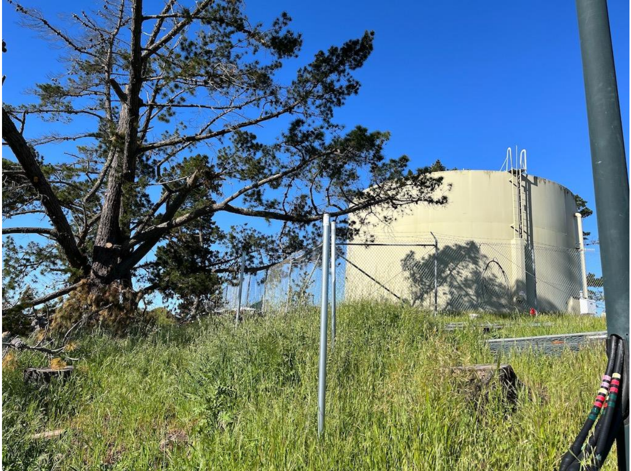
Figure 6. Existing Trees and Fencing, looking South.
