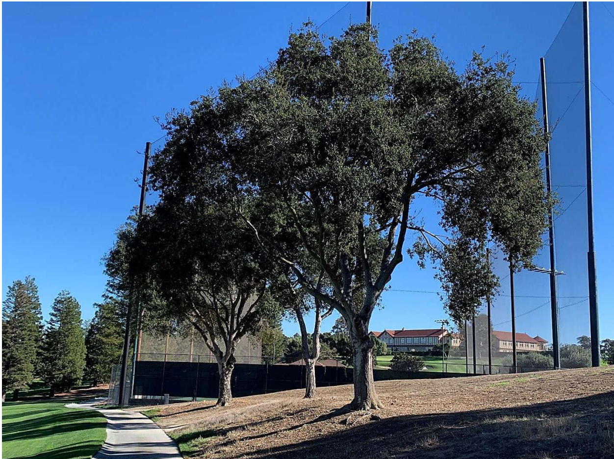
Image #1 – Project site looking west. Trees T1, T2 and T3, coast live oak, left to right.
