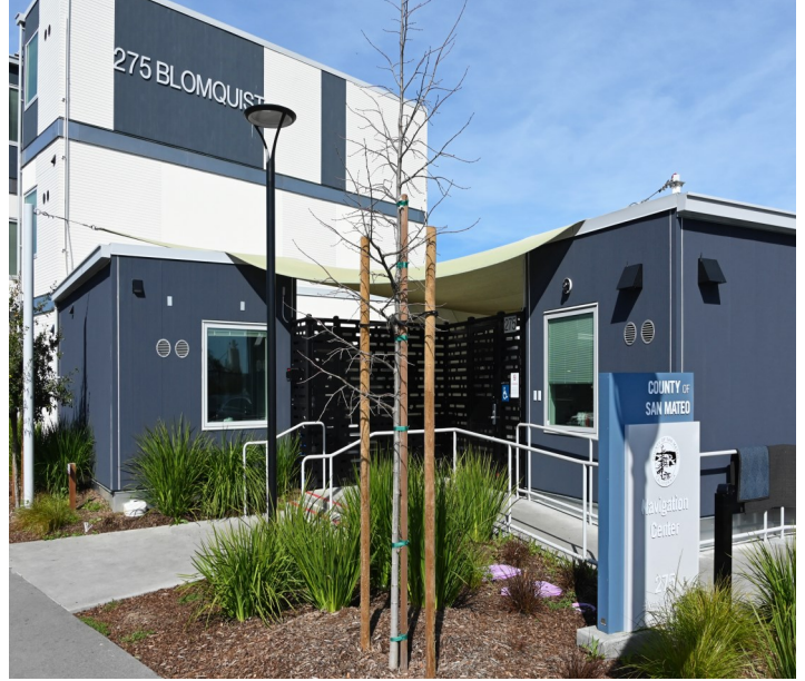
Navigation Center for shelter and housing services © County of San Mateo
