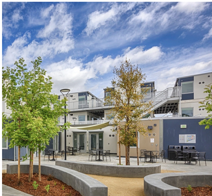
Navigation Center for shelter and housing services © County of San Mateo
