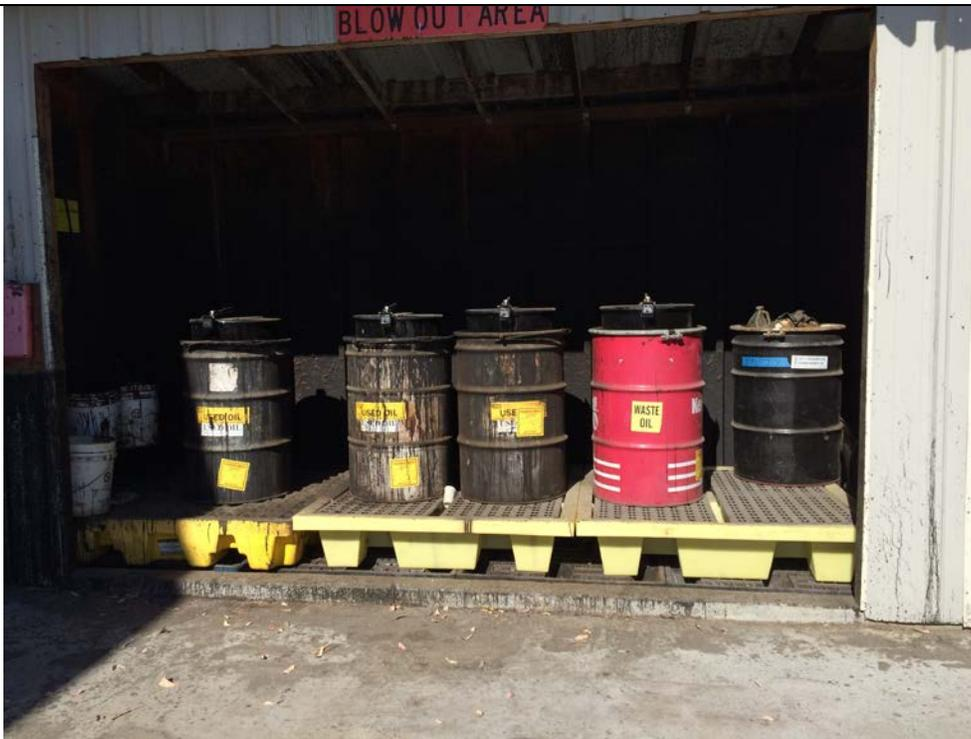
Photo 8: Oil Blow-Out Area containing five 55-gallon drums on secondary containment.
