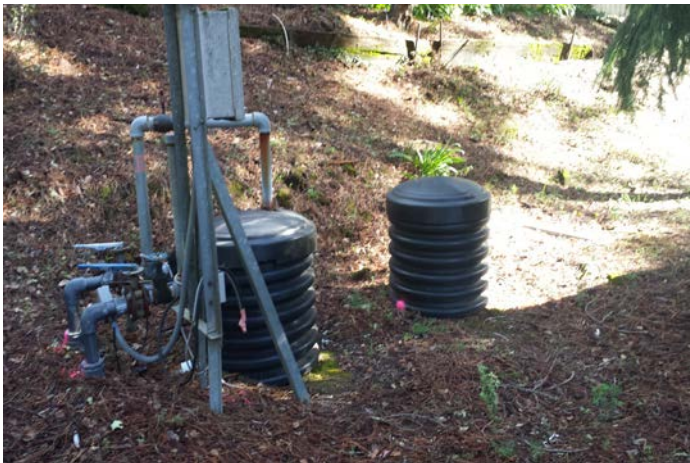
Photo 5: View of septic system area.
