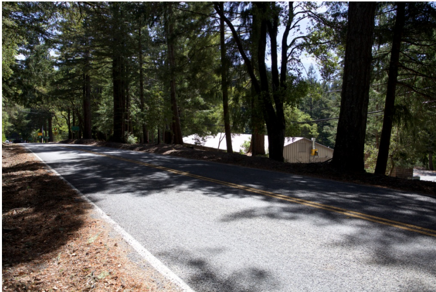
Photograph 16: View of apparatus building roof from Skyline Boulevard (looking south/southwest). The new driveway entrance would be past the apparatus building.
