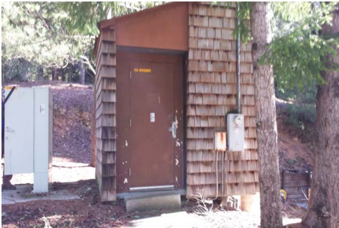
Photo 3: View of AT&T Communication shed onsite.
