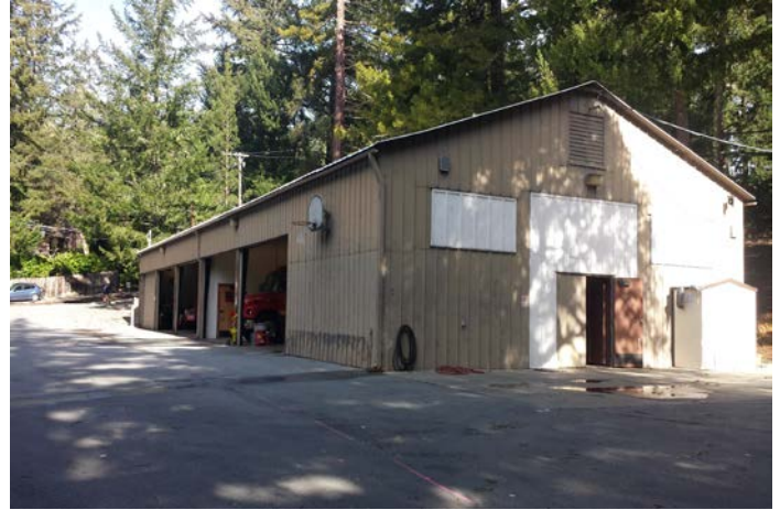
Photo 2: View of Apparatus Building.
