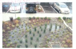
Bioretention areas function as soil and plantbased filtration devices that remove pollutants through a variety of physical, biological, and chemical treatment processes. These facilities normally consist of a grass buffer strip, sand bed, ponding area, organic layer or mulch layer, planting soil, and plants.
