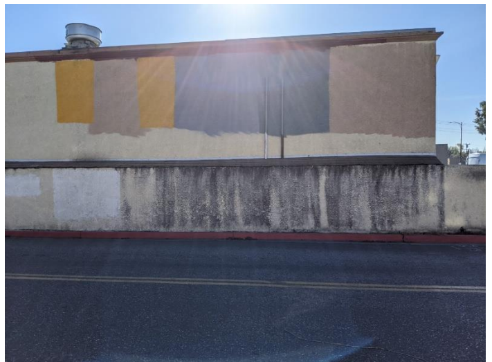
ADJACENT PROPERTY TO THE SOUTH (CONVENIENCE STORE MARKET)
